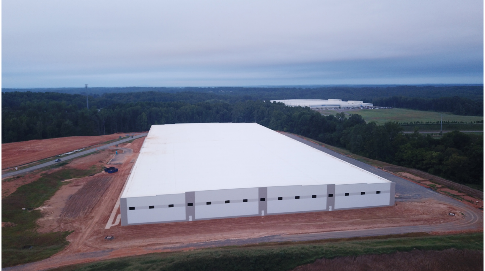
Davie Industrial Center Building 1 - Ready for Upfit
