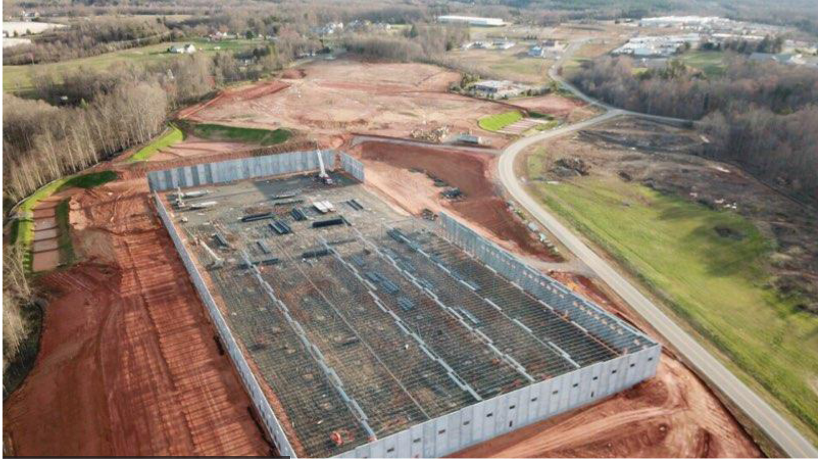
Davie Industrial Center Building 1 - Pad Underway
