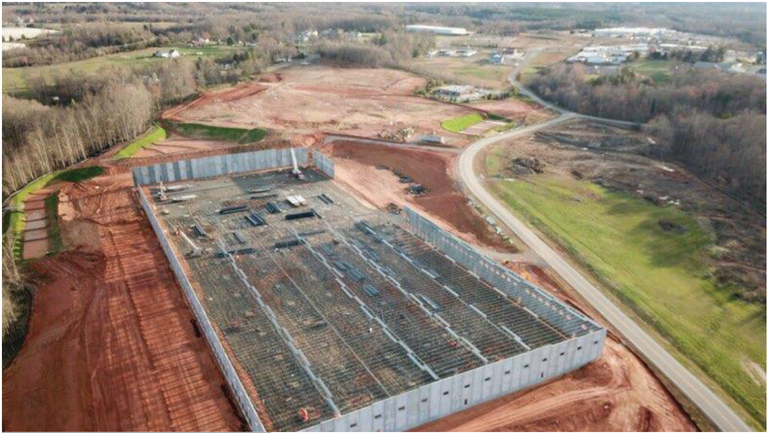
Davie Industrial Center Building 1 - Under Construction
