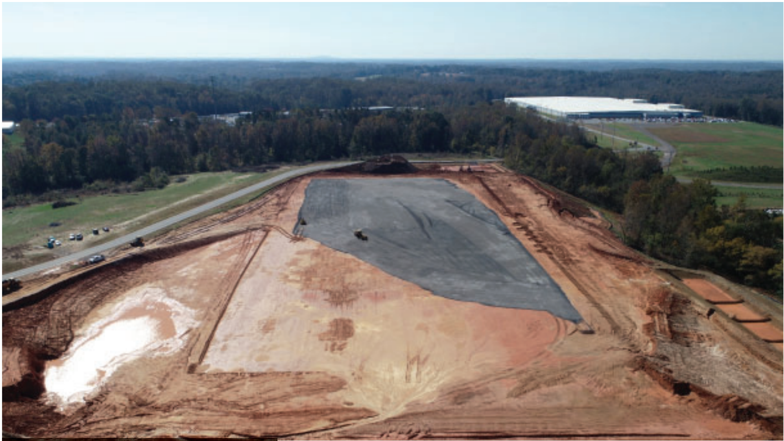
Davie Industrial Center Building 1 - Pad Underway
